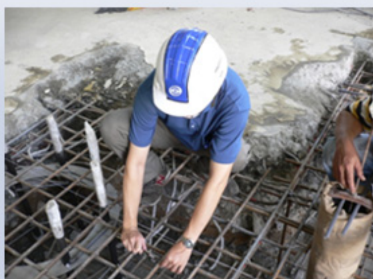
YV1200 Reinforcing bar binding inspection for foundation pit
